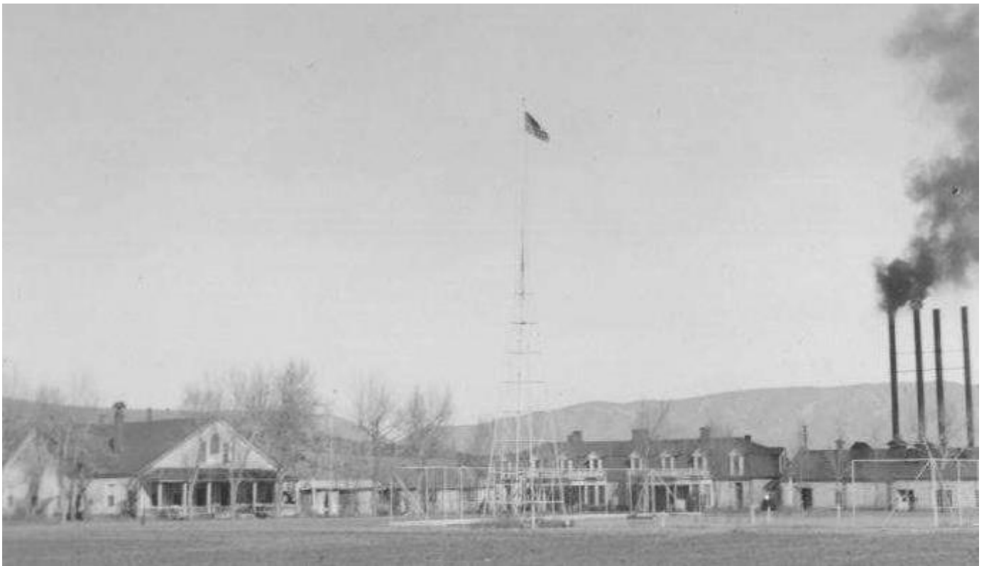
Bldg. 3 is at left, with Bldg. No. 4 and the old power plant at right.
