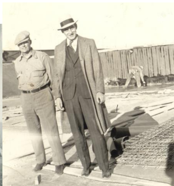
Ed White, left, at construction site of new plant
