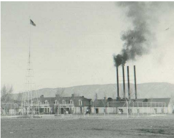
Old power plant next to Bldg. No. 4
