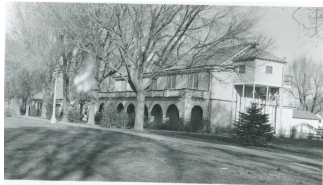
The Amusement Building plainly showing the projection booth added to the second floor.
