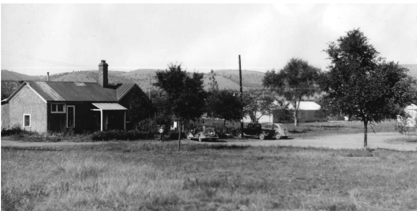
Bldg. 15, Engineer's House, Willett White in yard.
